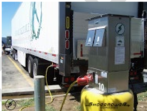
Figure III.A-4: Parking Area Power Plug Pedestal
