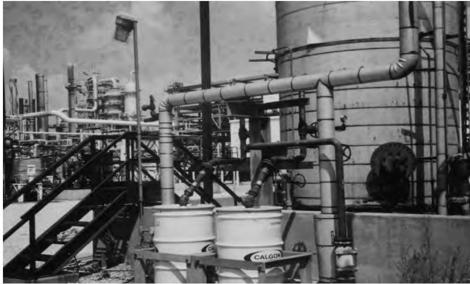
Figure XI-4: Use of Carbon Adsorption for Control of Wastewater Collection Systems at a Petroleum Refinery
