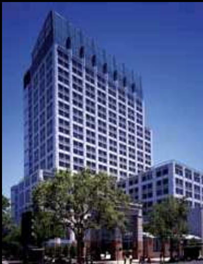
Cal/EPA Headquarters Sacramento, CA Energy savings add up to ~ $1.5 million a year (LEED EB platinum certified)
